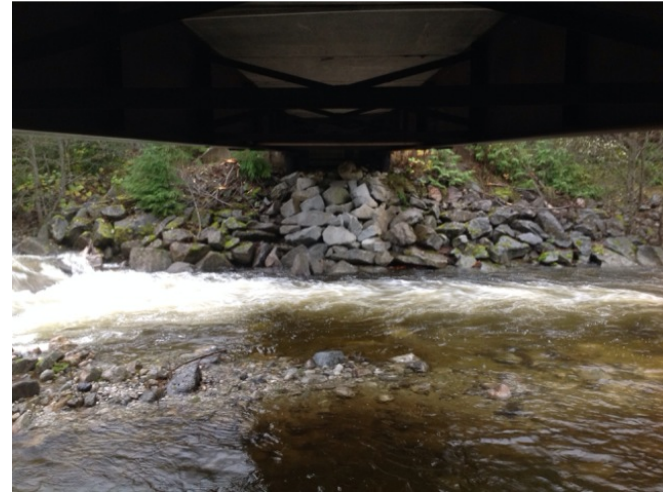
Left Bank Abutment when facing downstream
