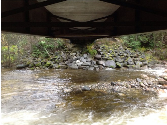
Right Bank Abutment when facing downstream
