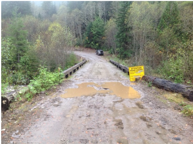
Approach from Right Bank when facing downstream
