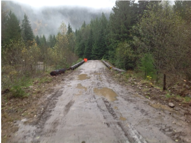
Approach from Left Bank when facing downstream
